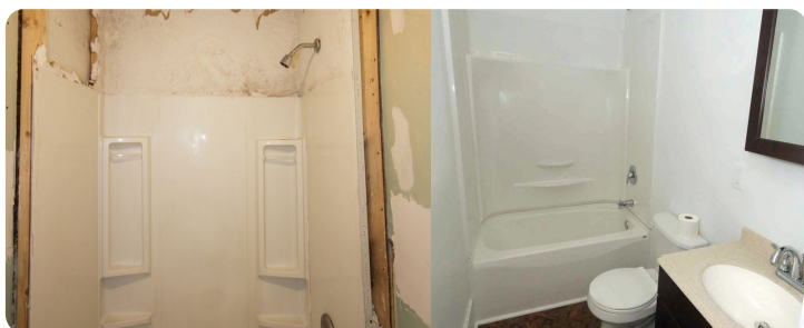
Before & After: Full Bath Renovation
